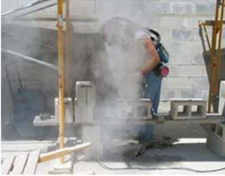
Cutting block without dust controls
