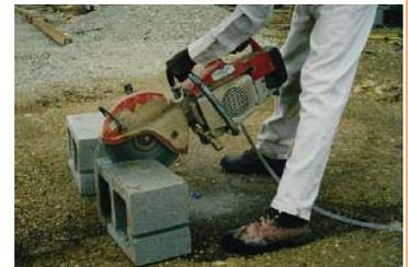
When applying water to the blade, exposures of handheld saw operators to silica are considerably reduced. Photo courtesy of OSHA.
