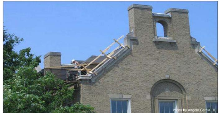
such as holes or skylights and leading edges, then plan and select fall protection suitable to that work, such as personal fall arrest systems (PFAS).
