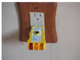
"Open ground" means that the ground wire has not been properly connected. A simple electrical tester should be used to check outlets to ensure proper wiring.
